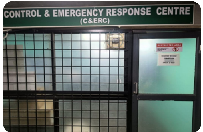
Control & Emergency Response Centre
